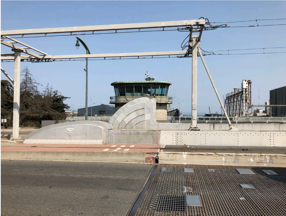
Deteriorated open grid decking and sidewalk grates – requires ongoing spot repairs and poses a safety hazard
