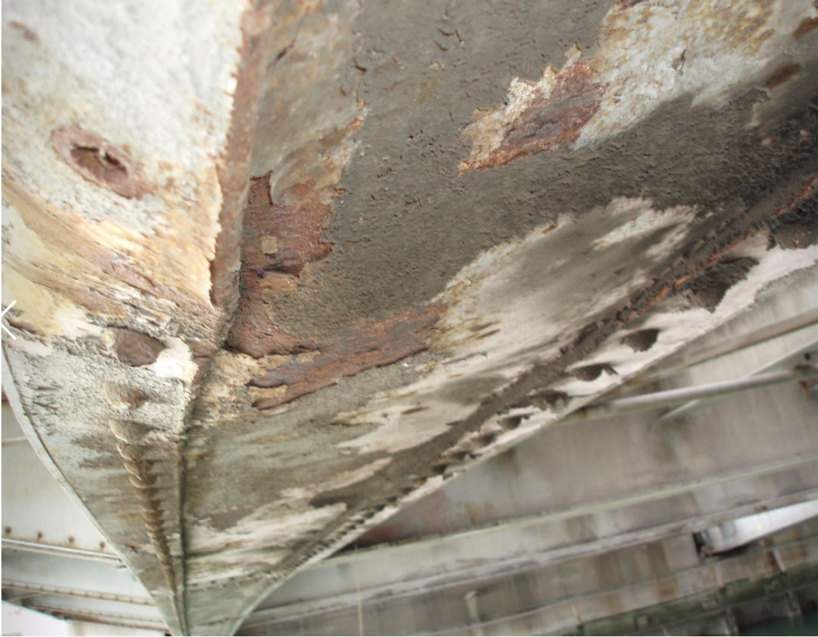
Deteriorated girders and fatigue cracks – Structural deficiencies noted in Caltrans Bridge Inspection – Impetus for rehabilitation in 2013
