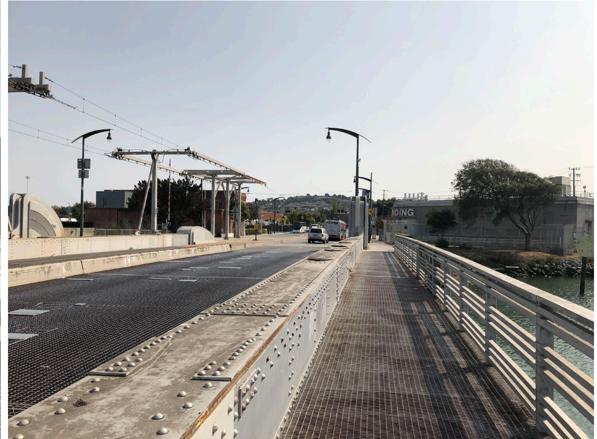
Deteriorated open grid decking and sidewalk grates – requires ongoing spot repairs and poses a safety hazard
